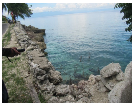
Penetrated seawalls noted along the coast of Barangay Guiwanon. Geographic coordinates N9°35'16.9" 123°18'52.9"E.
