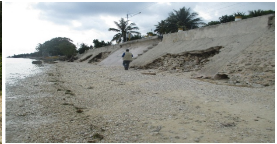
One of the breached seawalls observed along the coastline of Oslob, Cebu. Photo above is located at Brgy. Lagunde with geographic coordinates 9° 31' 55.0" N / 123° 26' 16.8" E.
